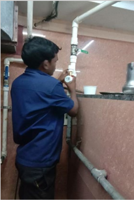
Smart water meter installed, tap for vessel / plate washing without bubble90 and with BS6 (Metal) bubble90 at Mc Donalds
